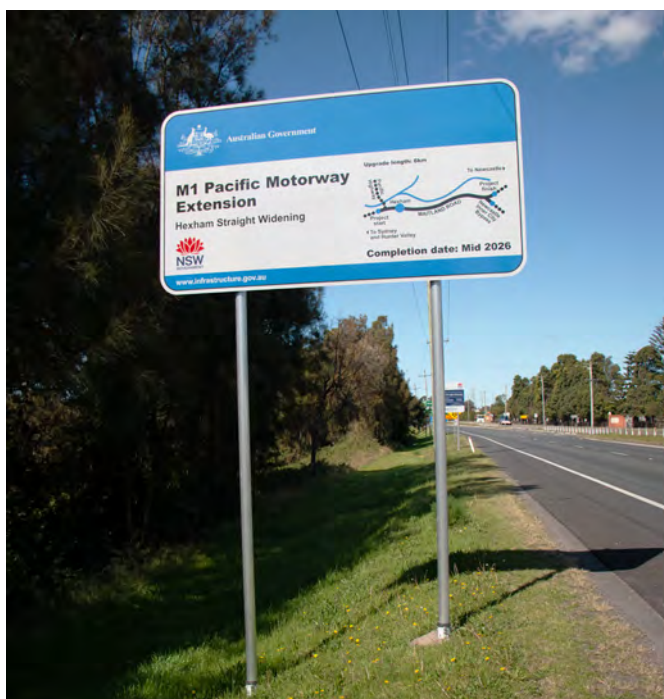
Signfix frangible poles range 60-114mm in outer diameter and hold up to 16m 2 road signs in Australian wind regions.
